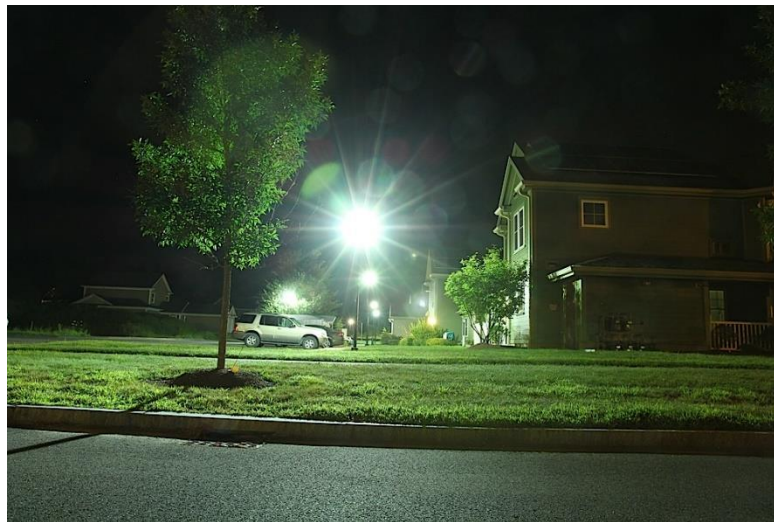
Figure 2: Example of glare from a light pole
