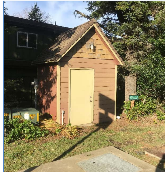
Figure 4-21 | Intertie Pump Station on Highway 101
