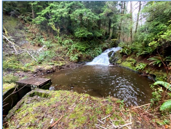
Figure 4-4| Salmon Creek Intake
