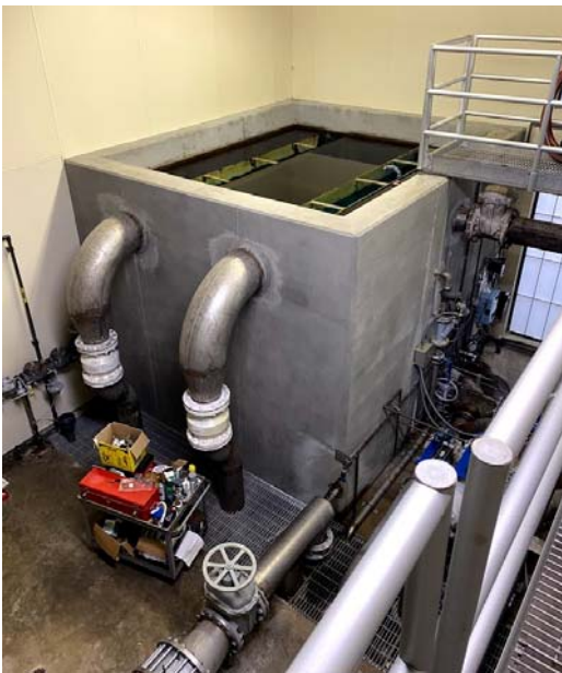
Figure 4-8 | Mixed-media Filters
