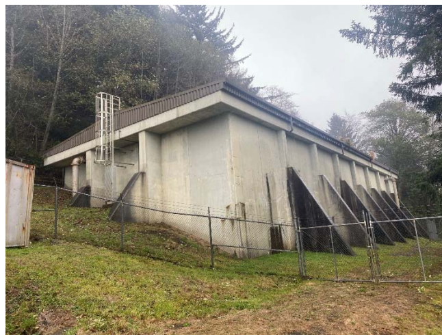
Figure 4-10 | Upper Radar Road Reservoir
