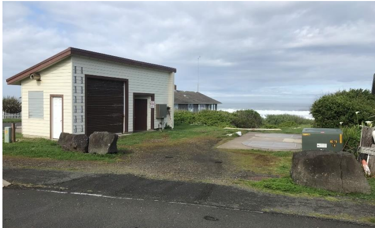
Figure 4-5 Main Pump Station
