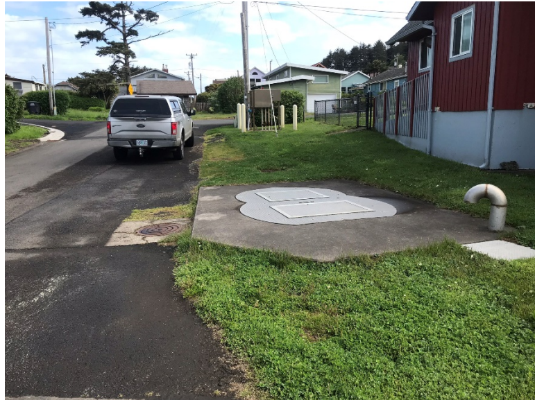
Figure 4-8 Pontiac Pump Station
