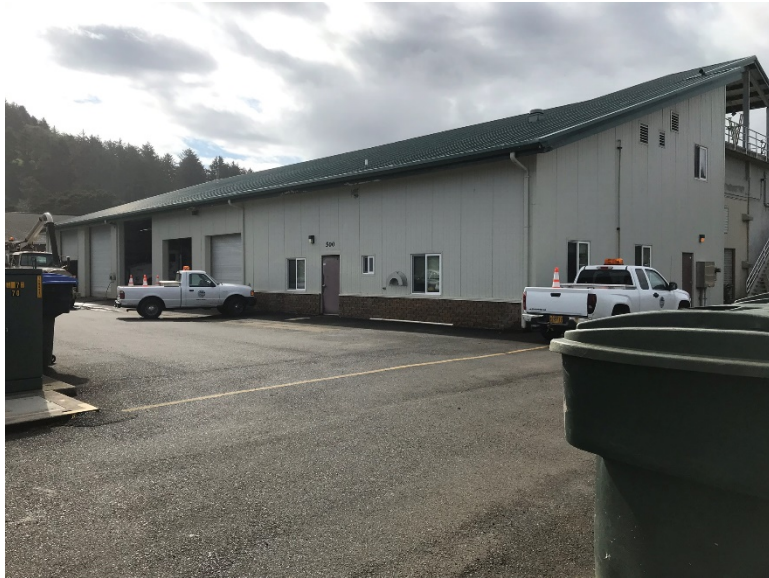
Figure 4-25 Public Works Building
