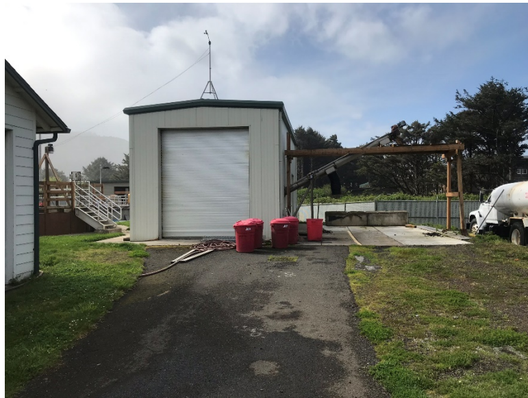
Figure 4-22 Solids Handling Building
