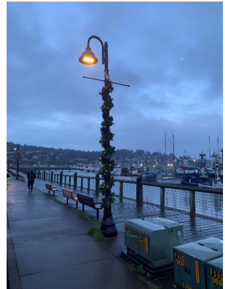
CLPUD DECORATIVE DOWNCAST LIGHT NEWPORT BAY BOULEVARD BOARDWALK
