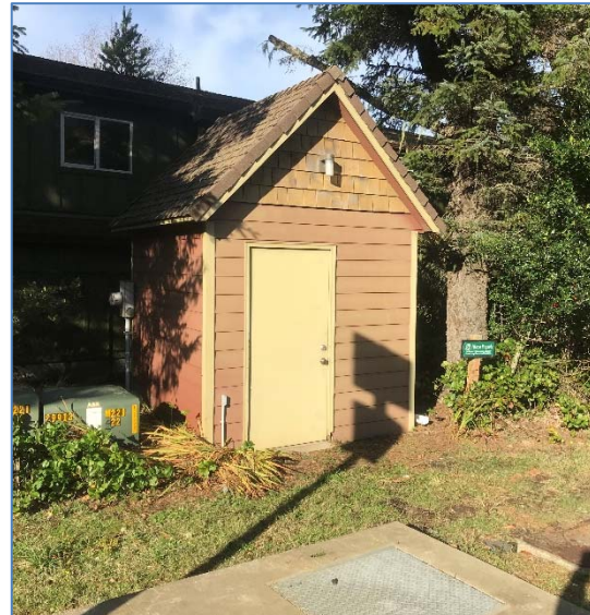
Figure 4-21 | Intertie Pump Station on Highway 101
