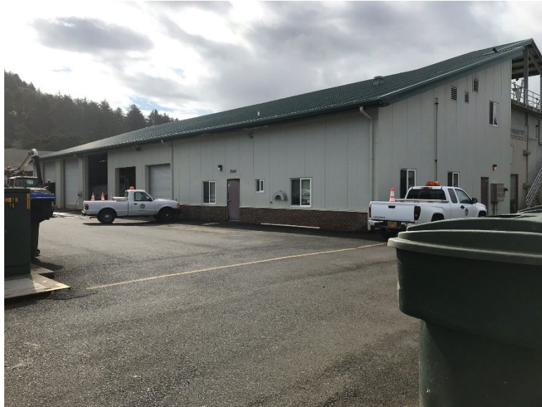
Figure 4-25 | Public Works Building
