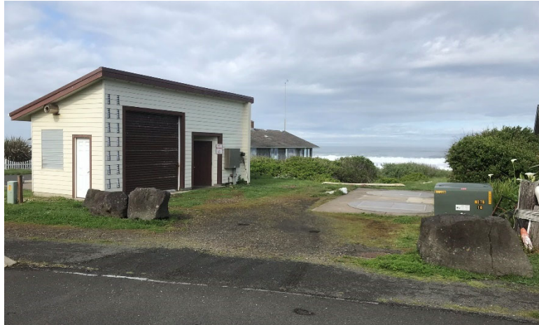
Figure 4-5 | Main Pump Station
