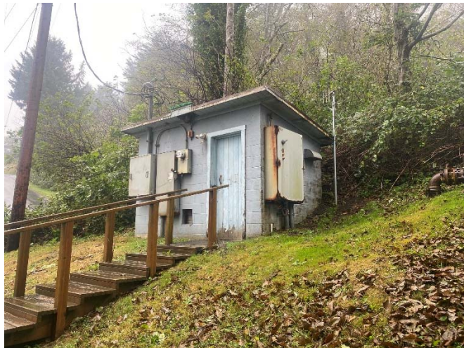
Figure 4-16 | Radar Road Pump Station
