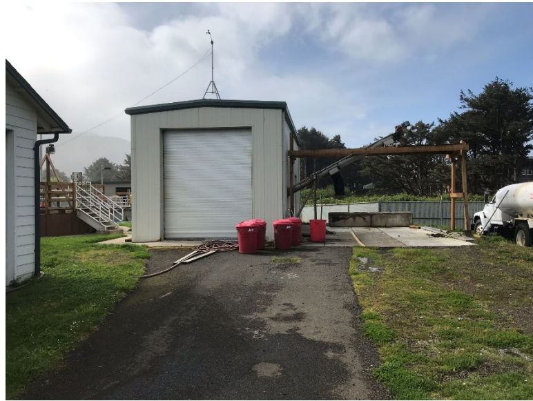
Figure 4-22 | Solids Handling Building
