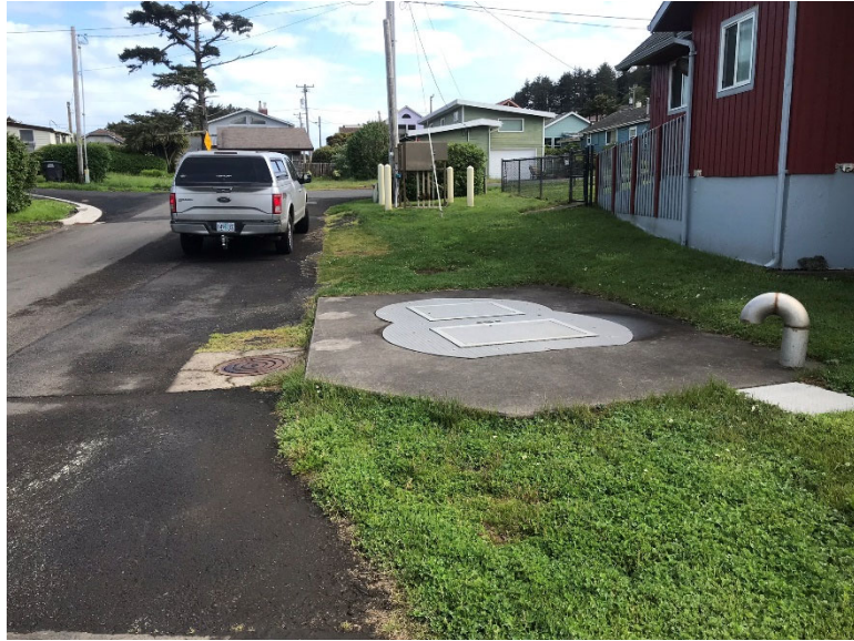
Figure 4-8 | Pontiac Pump Station
