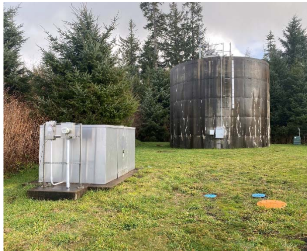
Figure 4-20 | Upper Blackstone Pump Station & Reservoir
