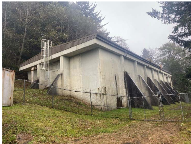
Figure 4-10 | Upper Radar Road Reservoir
