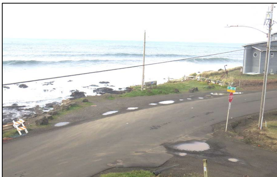
Figure 6. Photo showing the current gravelled lot at Ocean View Drive and 6 th Street.
