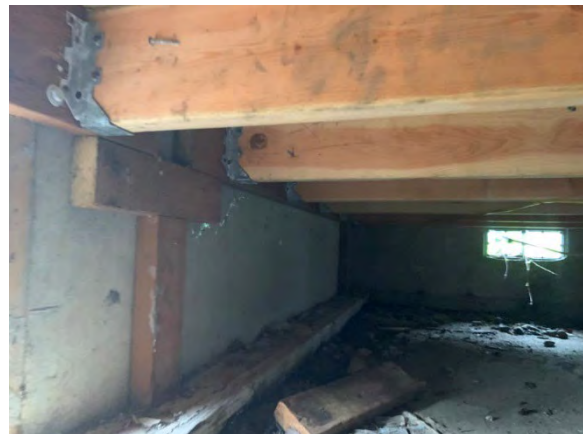
Figure 9 - BATHROOM ADDITION FOUNDATION AND FLOOR SUPPORT
