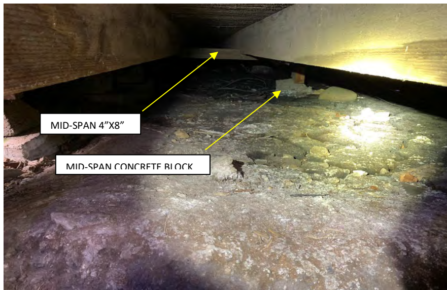
Figure 3- CIP CONCRETE BLOCK FOOTING - N to S MID-SPAN, FACING WEST
