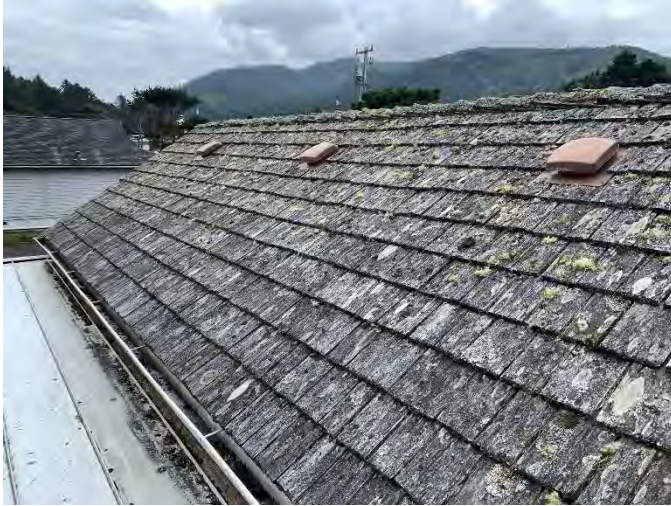
Figure 12- MUSEUM CEDAR SHAKE ROOF
