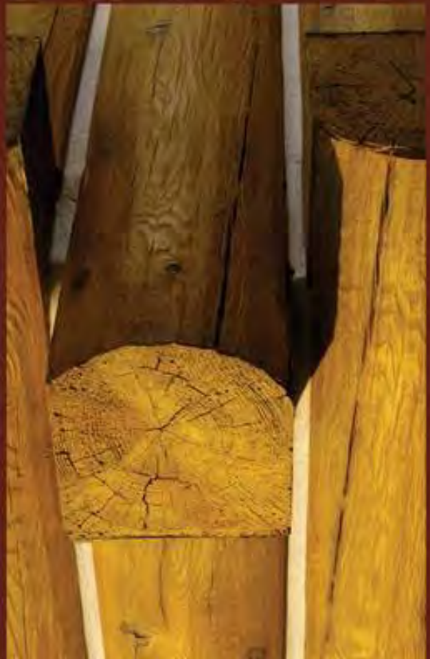
16" HAND-HEWN EVERLOGS™ (SADDLE NOTCH CORNER)
