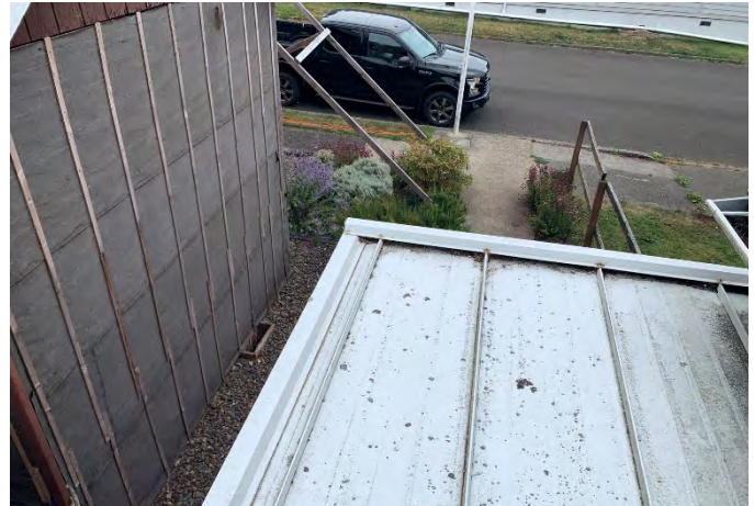
Figure 14- ENTRYWAY/BATHROOM STANDING SEAM METAL ROOF
