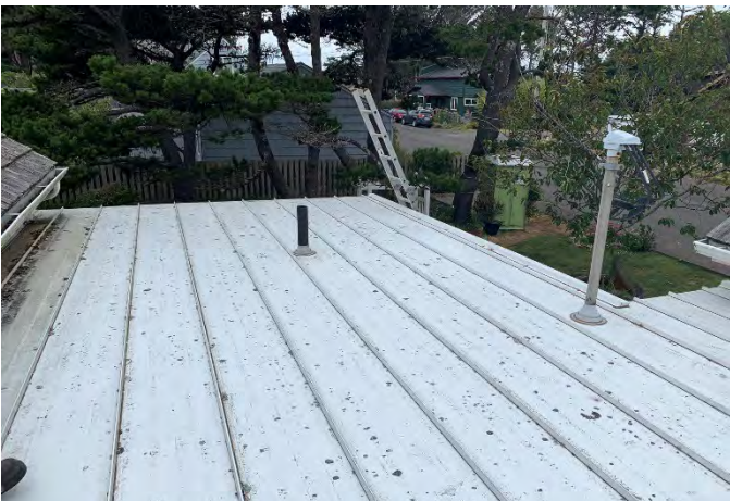
Figure 14- ENTRYWAY/BATHROOM STANDING SEAM METAL ROOF
