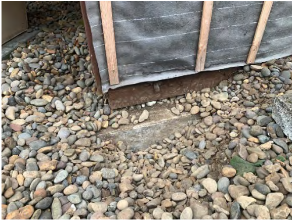
Figure 4 -CIP CONCRETE BLOCK FOOTING - NE CORNER
