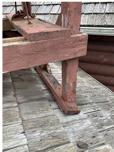
Figure 15- BELL TOWER CONNECTION TO VESTIBULE ROOF
