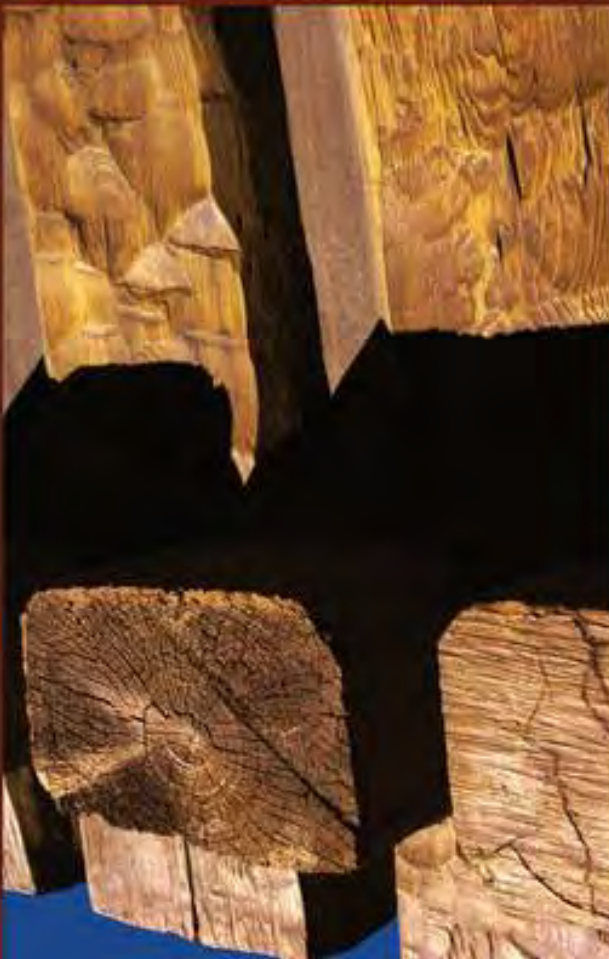
16" HAND-HEWN EVERLOGS™ (SADDLE NOTCH CORNER)
