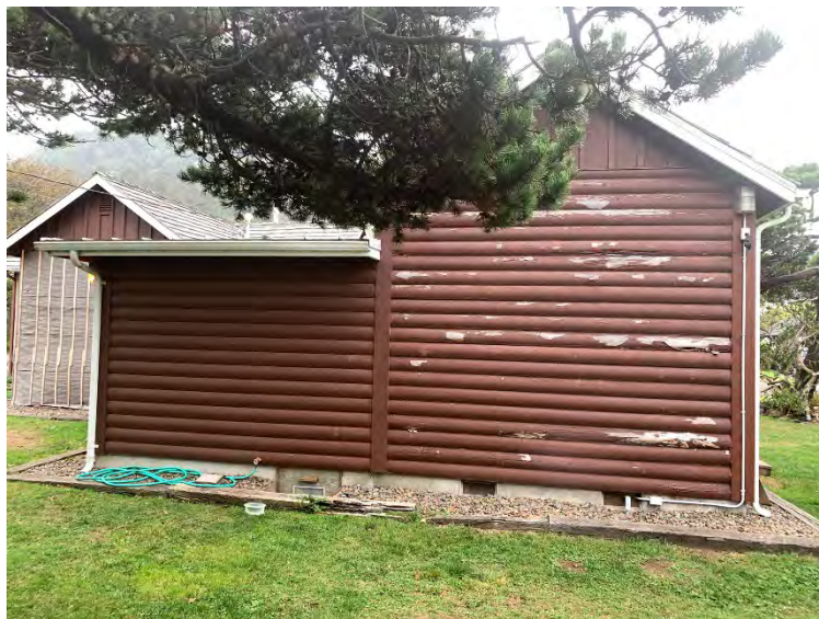
Figure 17- TRANSITION BETWEEN BATHROOM AND MUSEUM ADDITIONS
