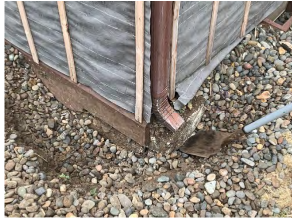
Figure 5 - CIP CONCRETE BLOCK FOOTING - NW CORNER
