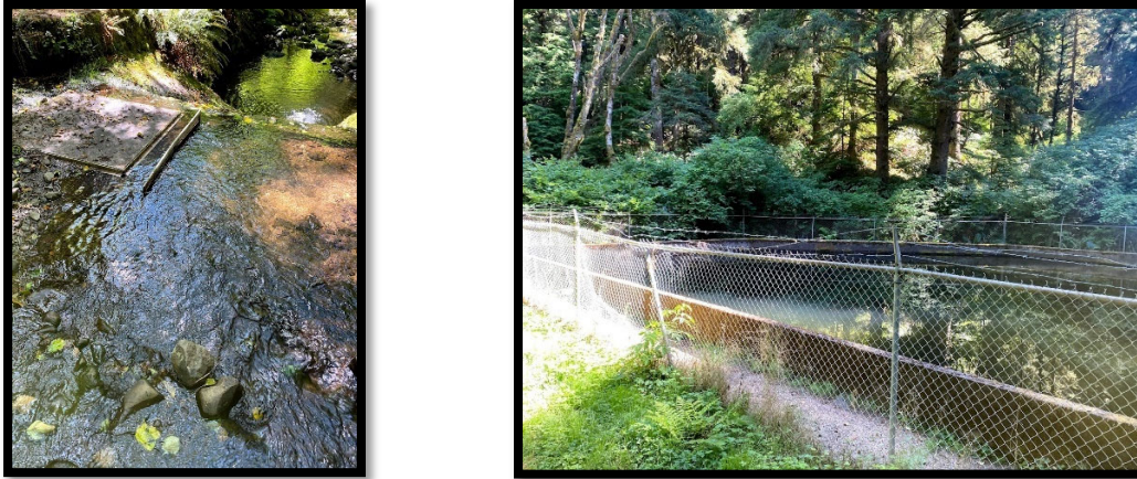
FIGURE 2.5 – BIG CREEK INTAKE AND SETTLING BASIN
