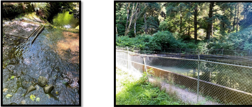
FIGURE 2.5 – BIG CREEK INTAKE AND SETTLING BASIN
