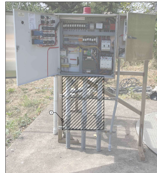
2 RIVERSIDE PS DEMOLITION PHOTO SCALE: NTS
