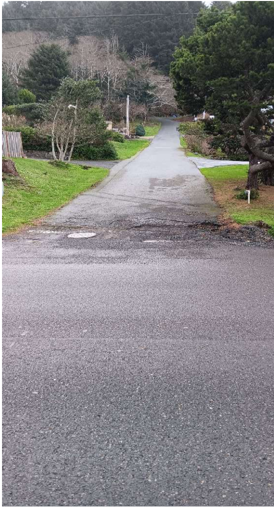
South Reeves Circle @ Hwy 101 S:
