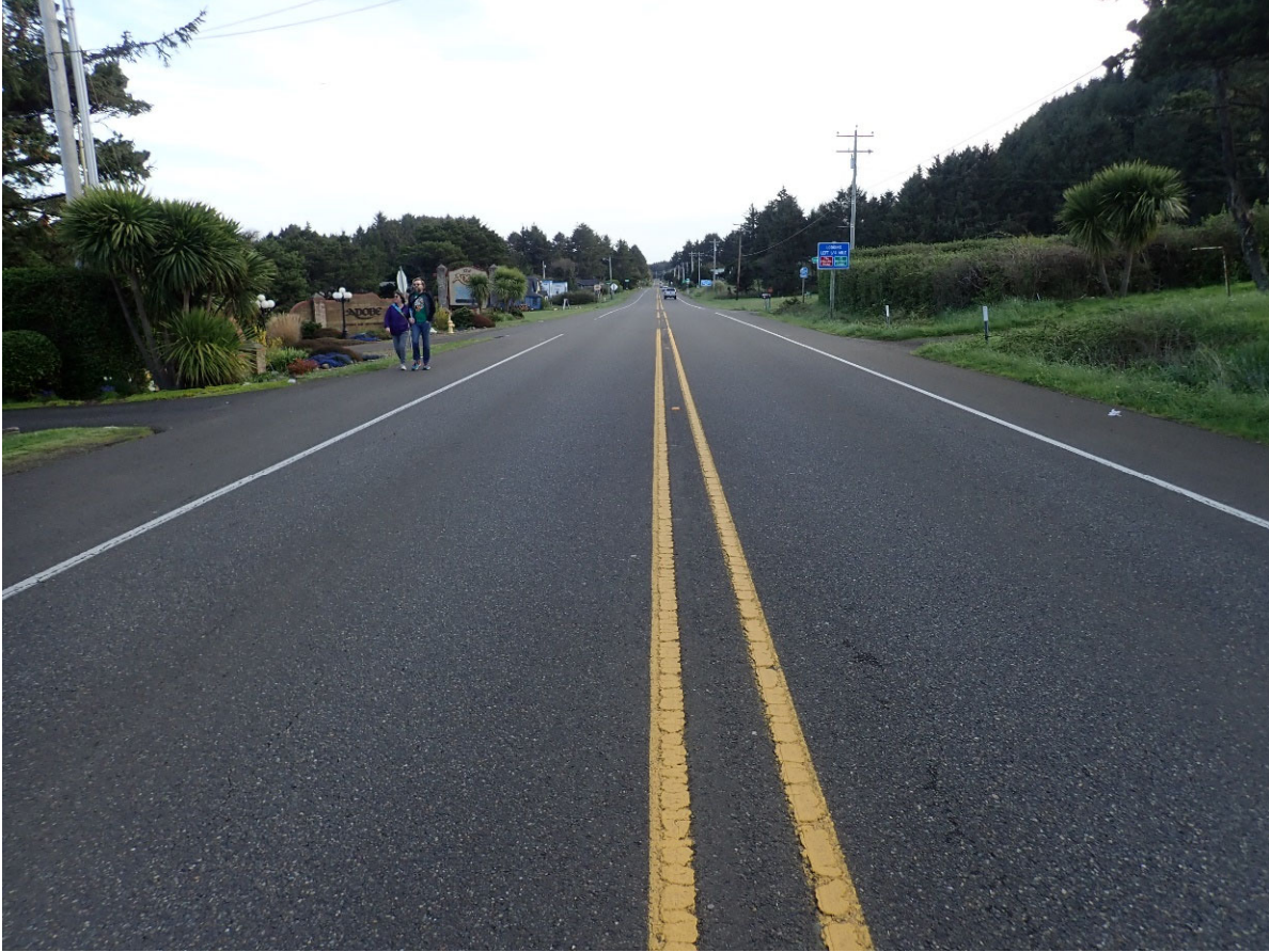
7. Looking northbound from 75 feet north of Aqua Vista Loop (northern conn.).
