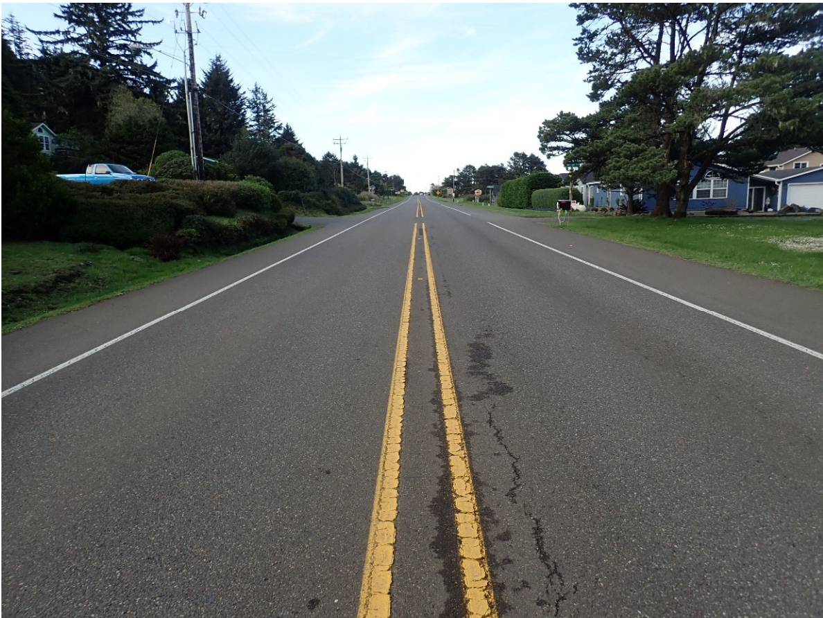
6. Looking southbound from 130 feet north of Coolidge Lane.
