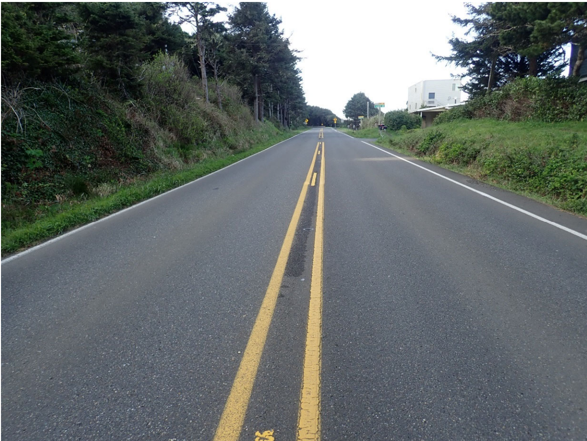
22. Looking southbound from 150 feet south of Windy Way.
