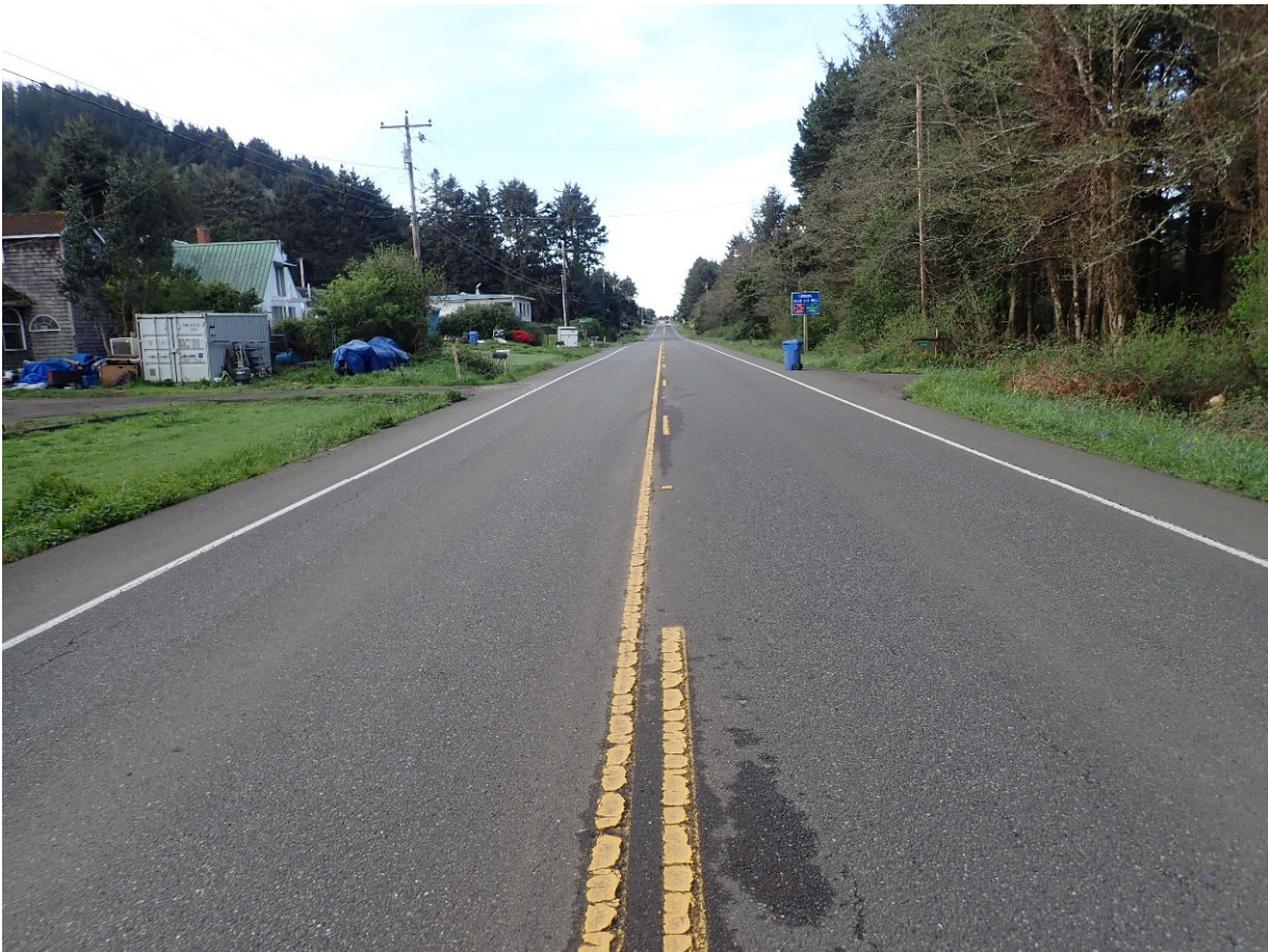
2. Looking southbound from 400 feet south of Trout Street.
