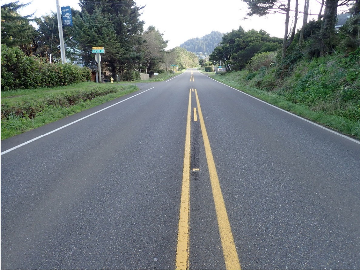
21. Looking northbound from 150 feet south of Windy Way.
