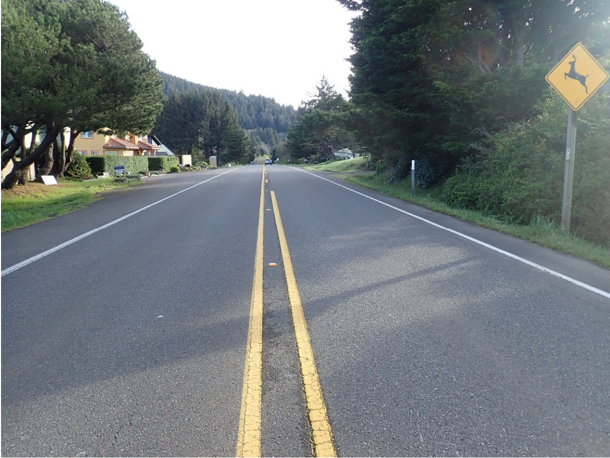
15. Looking northbound from 100 feet north of Reeves Circle (northern conn.).
