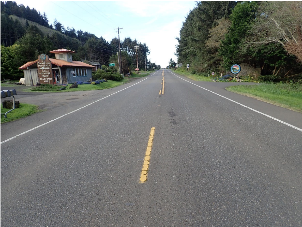
4. Looking southbound from 200 feet north of Ocean Wayside Lane.
